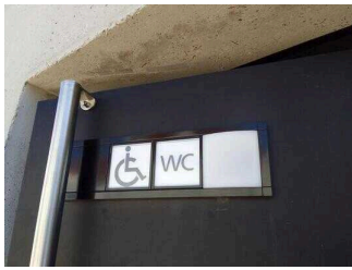
WC in the forecourt area
