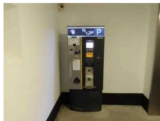
Parking machine in the underground garage
